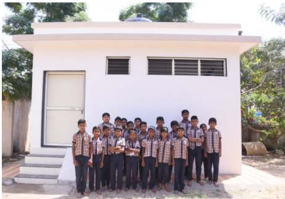
After Construction of toilets for boys at a primary school in Abrama, Valsad
